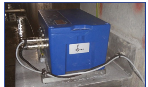
Dam Station — a high humidity area.
